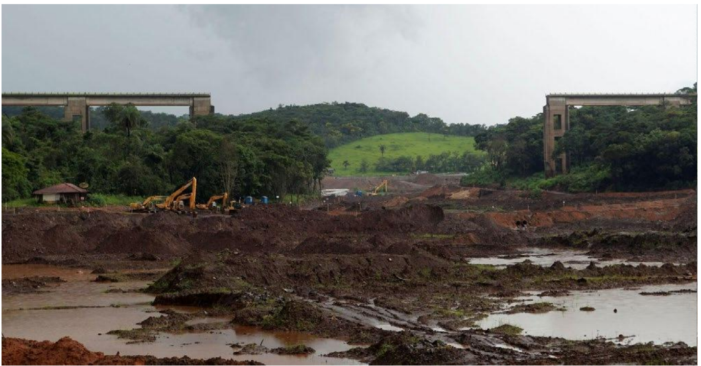
Vale's tailings dam in Brumadinho
